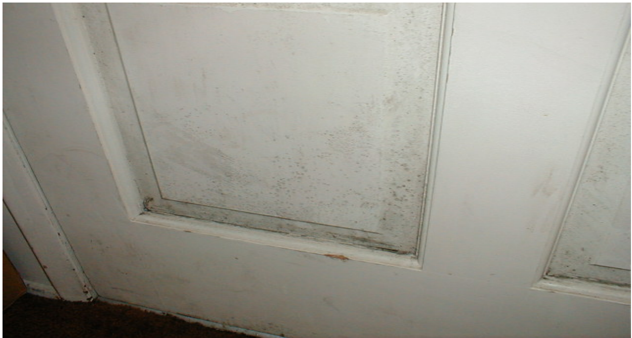
Figure 6. Condensation: Mold growth on inside surface of exterior door. Again, cold surface meets moist air, gets wet and supports mold growth. This can be washed off and repainted.
