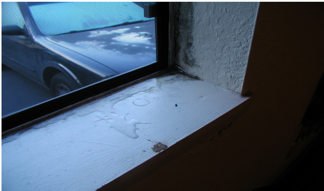
Figure 1. Condensation from excessive indoor moisture on the window glass drained and ponded on the window sill, soaked into and wicked up the drywall, and provided plenty of moisture to cause the black mold growth visible next to the window.
