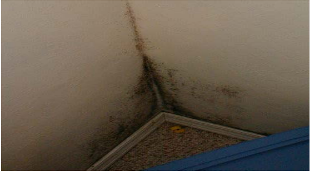
Figure 5. Condensation: Mold growth in bedroom corner of exterior wall. The combination of high relative humidity from occupants breathing all night (exhaling water vapor) and the cool surfaces of the exterior wall led to condensation and mold growth.
