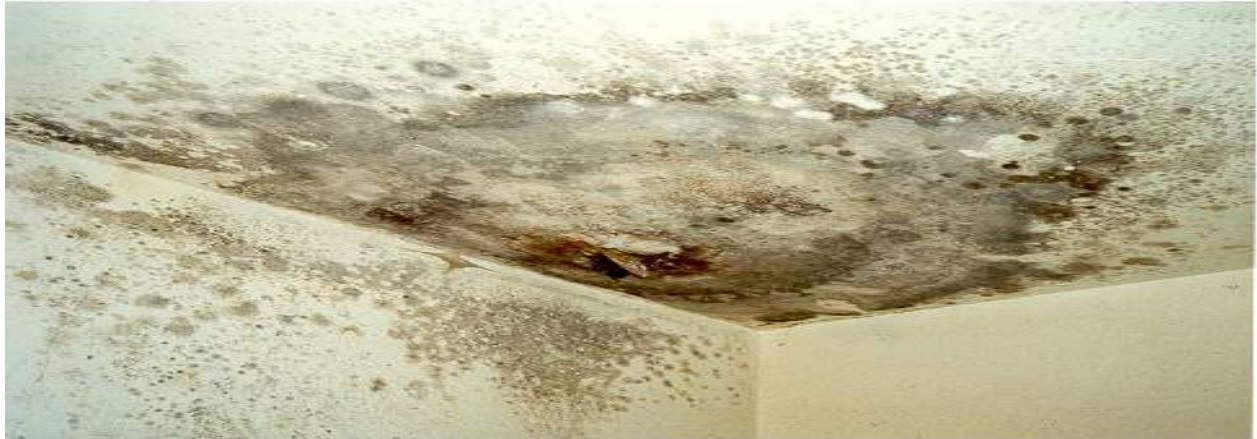
Figure 10. Leak from roof or plumbing: Left unrepaired, a small leak can become a big problem. This wallboard must be removed using personal protection and a plastic enclosure under negative pressure exhausted to outside to prevent further contamination of occupant property. The ceiling and wall cavities will also be moldy and need careful cleaning by protected workers.
