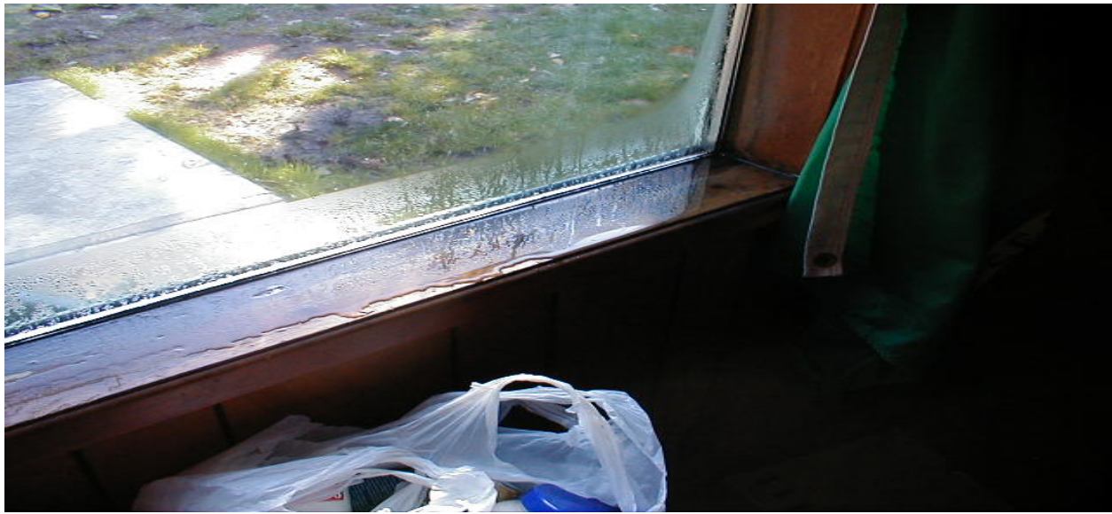
Figure 2. Too much moisture in the air (high relative humidity) leads to unwanted condensation on cool surfaces like double pane windows in cold weather. The moisture drips down, accumulates on sills, and can leak into wall cavities below causing hidden mold growth on wood and paper backed wallboard. Single pane windows will be colder still, resulting in condensation even with normal indoor humidity levels (below 40%) and may require daily drying of sills with towels to prevent mold growth and water damage.
